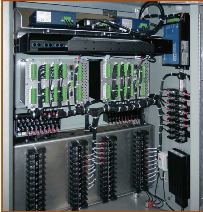
Two SEL-2411 Programmable Automation Controllers, two SEL-2725 Five-Port Ethernet Switches, SEL-9321 Low-Voltage DC Power Supply, SEL-2401 Satellite-Synchronized Clock, heater, fuses, terminal blocks, FT-1 switches, and a fiber patch panel in a dual-door cabinet.
