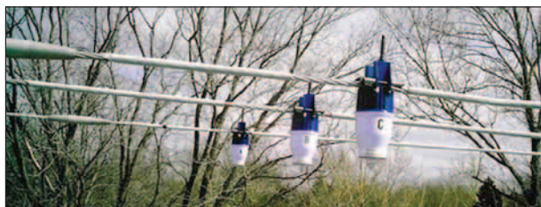
Wireless Sensor for Overhead Lines installation.
