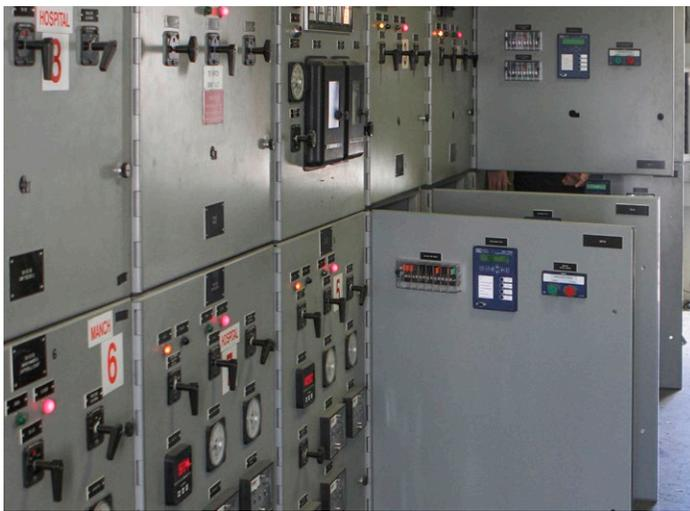
In many upgrades, just one or two digital relays can replace 20 or more EM relays and provide better protection.
