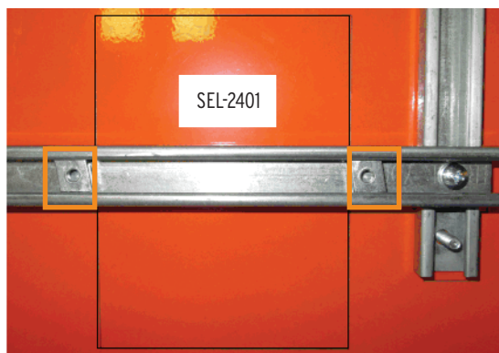
Figure 7 Install Channel Nuts
