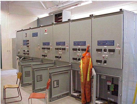
Figure 3—Shown above are SEL-351A Relays for feeder protection, SEL-351-7 Relays for the main incoming breaker, and the SEL-2030 Communications Processor as the central data collector. Larger stations may also have an SEL-387-5 Relay for differential protection.
