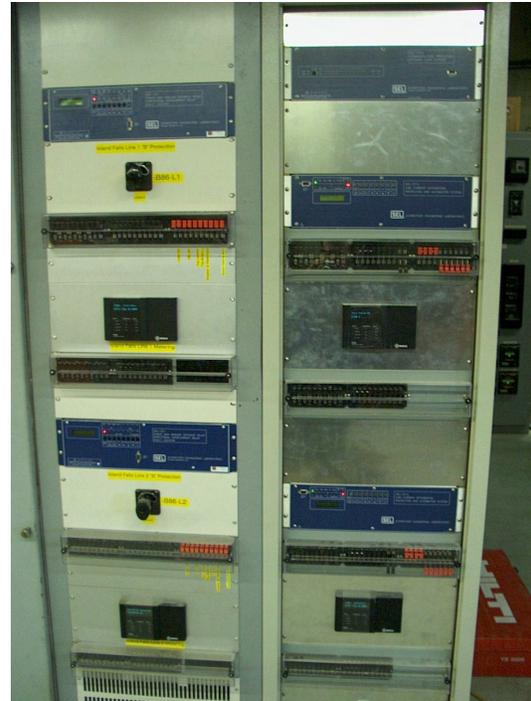
*Figure 3—The Iroquois Falls mill protection system utilizes GPS-synchronized time and the Ethernet LAN to communicate records, data, and Sequential Events Recorder files from the SEL relays. This exact information is used for reconstruction and analysis of events.*
