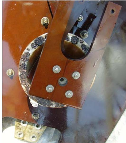
Figure 3—Inspection of the utility transformer revealed the damage caused to the rotor assembly (shown above) and the rotor of the tap changer (shown below) caused by arcing.
