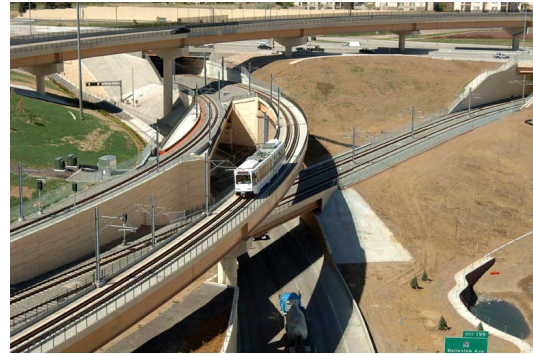
Figure 1—Shown above is the Denver Light Rail Transit System passenger train on the I-25/I-225 interchange. It has a light frame and small body that enable it to operate along crowded city streets and within tight urban corridors with frequent stops. Light rail was introduced to the region in 1994.
