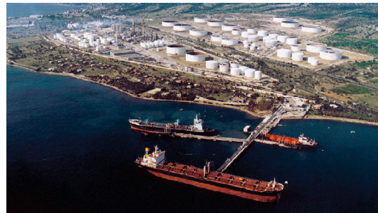
Figure 1—MOH is the largest privately held industrial complex in Greece and is one of the most modern refineries in Southeast Europe. Because of its flexibility, it can process crude oils of various characteristics and produce a full range of petroleum products. MOH complies with the most stringent international specifications and serves major petroleum marketing companies in Greece and abroad.
