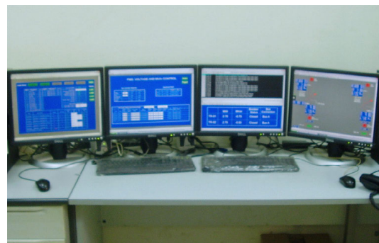
Figure 7—Remote-view stations used throughout the MOH plant allow for continuous visualization and diagnostics of the entire system.
