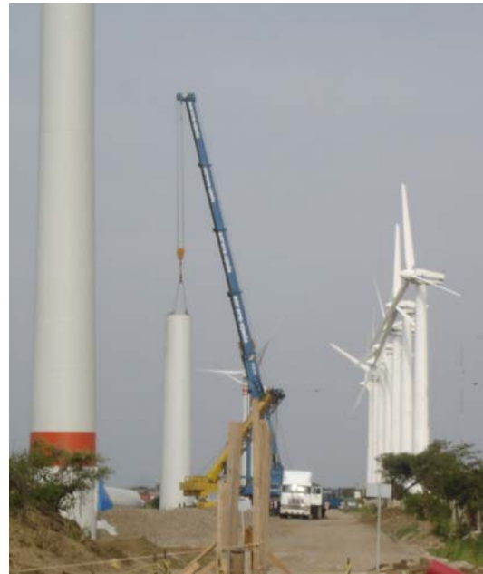
Figure 1—La Venta II wind farm during construction phase.
