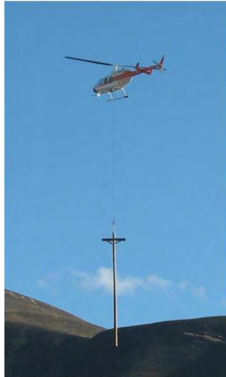
Figure 3—Some of the terrain in CPC’s service territory is so remote, a helicopter is used to place power poles when the cooperative builds new lines.
