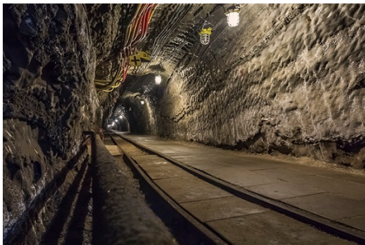
Figure 1—Typical Mine Interior
