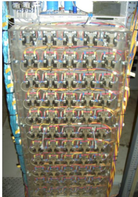
Figure 3 Using the Communications Processor's Multifunction Control Capabilities Eliminated all of the PLC Inputs, Control Outputs, and Interposing Relays Shown in These Two Photos
