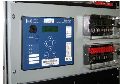
Fig. 4. Meter and Test Switches
