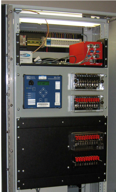
Fig. 3. Front View of New Dairyland Power Metering, Communications, and Automation Cabinet
