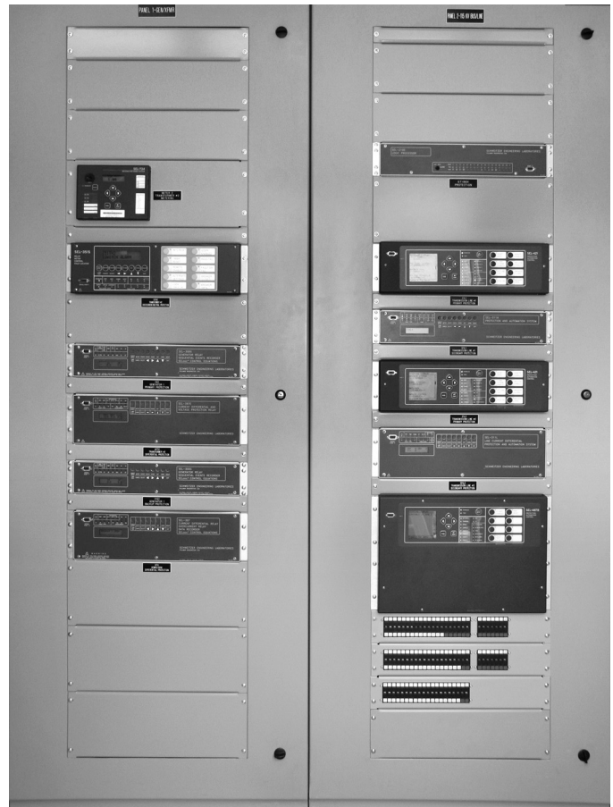
Fig. 6. Panels With Test Switches Designed Out
