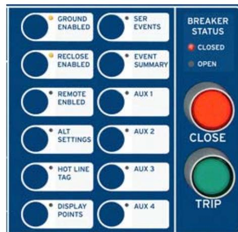
Fig. 11. Local Breaker Control Panel
