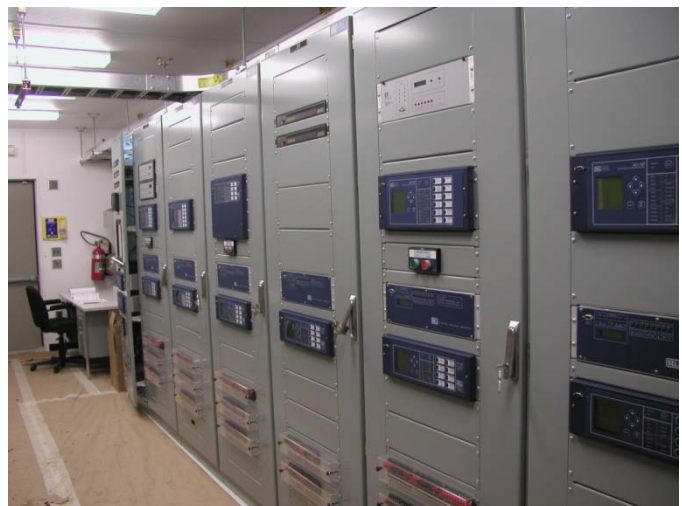
Fig. 6. A few smart and automated devices replace many discrete components
