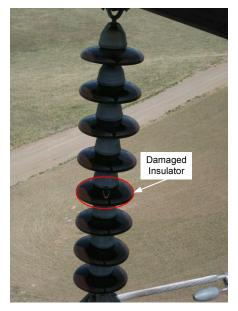
Fig. 26. Damaged insulator at 67.91 miles from Goshen terminal.
