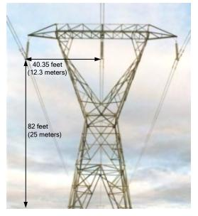
Fig. 5. Typical high-voltage transmission tower.
