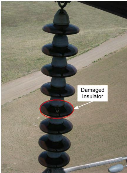
Fig. 26. Damaged insulator at 67.91 miles from Goshen terminal.
