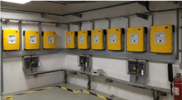
Fig. 5. Battery system inverters installed in the inverter room of the Guásimas del Metate solar farm. (Photo courtesy of Greenergy.)
