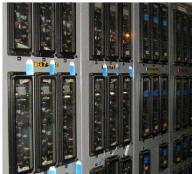
Figure 2. Electromechanical relay panel
