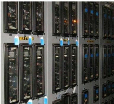
Figure 2. Electromechanical relay panel
