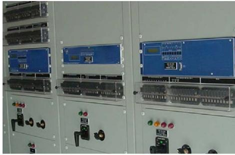
Figure 3. Microprocessor-based relay panel
