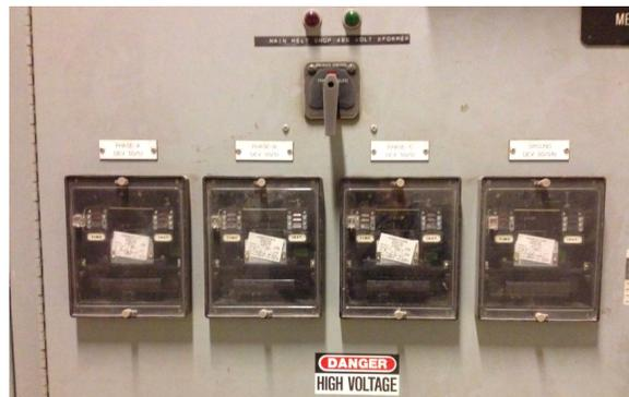
Figure 2. Original melt shop relay configuration (protecting only one circuit)
