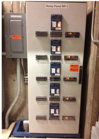
Figure 3. Melt shop switchgear relay panel (with complete protection for five circuits)
