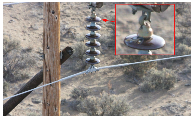
Fig. 12. Flashed-over insulator on the C-phase, tower 8/6 (eighth tower after the sixth mile) of the Brasada-Harney line.
