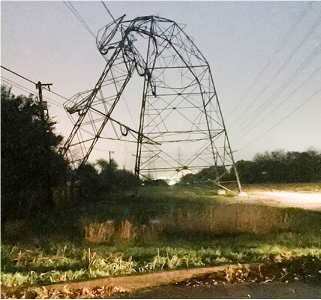
Fig. 1. High-voltage transmission tower damaged during storm
