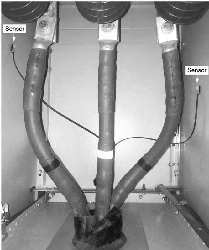
Fig. 12. Point Sensors Installed in Cable Compartment of 11 kV Outgoing Switchgear Panel
