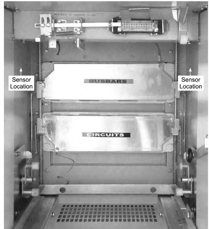
Fig. 11. Point Sensor Locations in Breaker Compartment of 11 kV Outgoing Switchgear Panel
