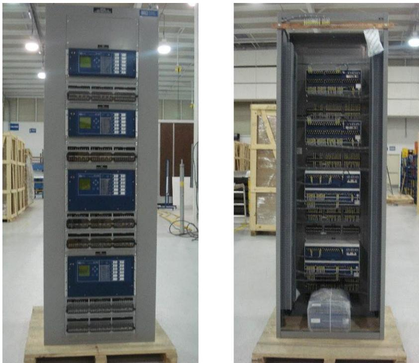
Figure 9 Example Transformer and Line Protection Relay Panel
